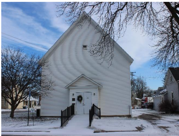
Finished Ramp with Railings Installed by Kem's Hardware
