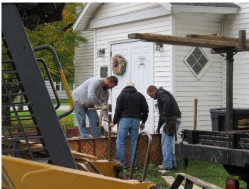
Crew from Wiggs Concrete Company Framing the Ramp
